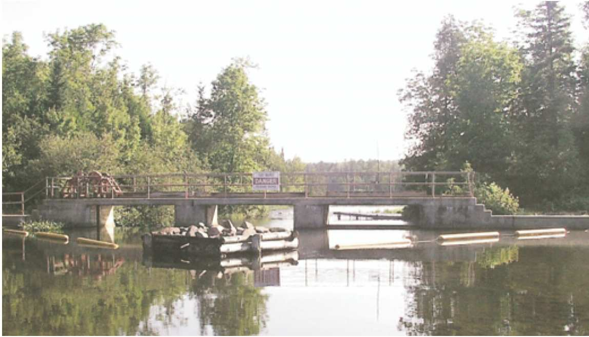
Photo #1 – Picture taken looking downstream from upstream of Turtle Dam
