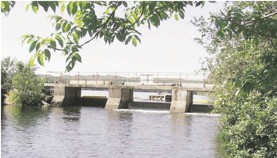
Photo #2 – Picture taken looking upstream from downstream of Turtle Dam
