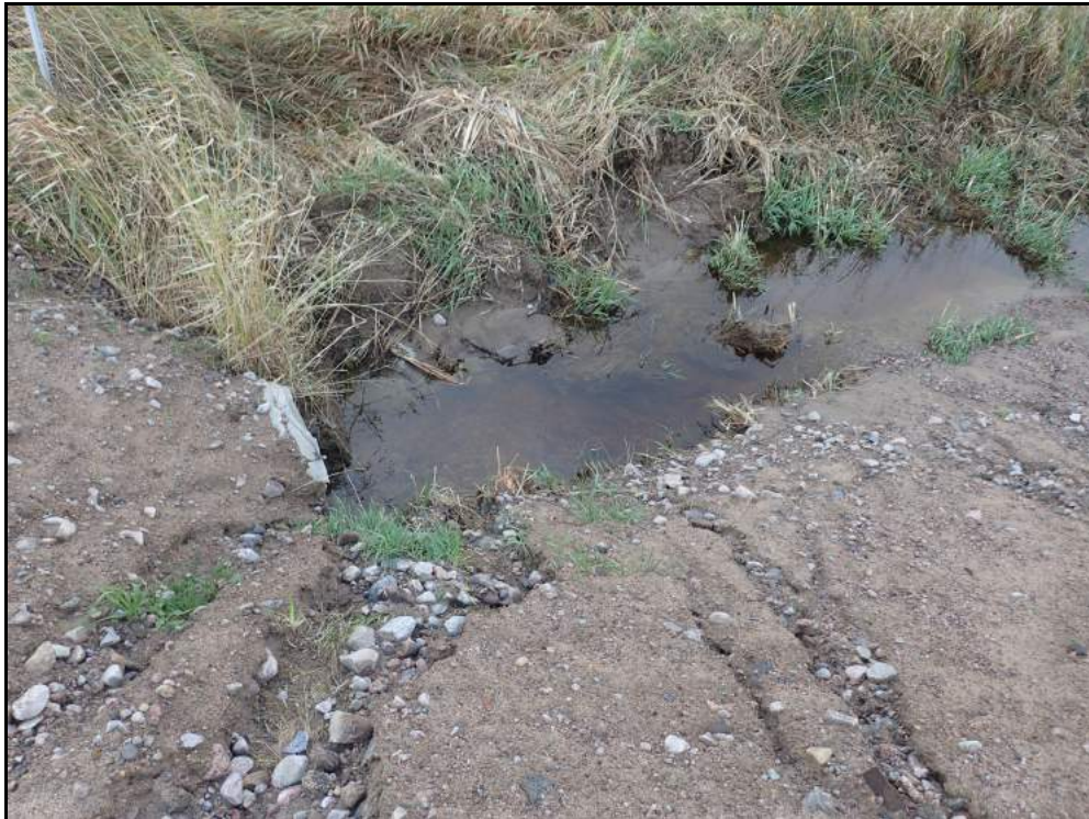
Figure 3.10: Rill erosion along road embankment – Graham Creek.
