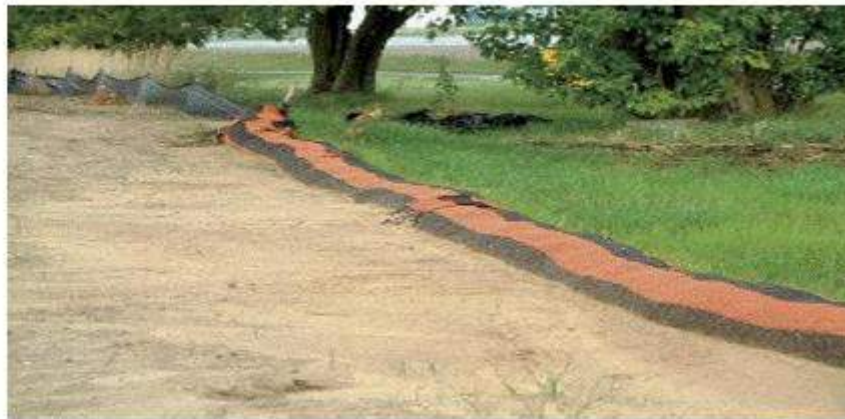
Example of Silt Soxx for Perimeter Control.
